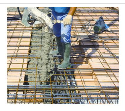
To construct a commercial building of such height required the very best superplasticiser available, as all concrete needs to be pumped, right up to level 80, some 259 metres above ground. The concrete also had to meet a slump range of 160 mm to 200 mm for different floor levels because of rebar interaction.
