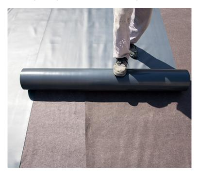
GCP Applied Technologies proposed BITUTHENE®3000HC, an adhesive membrane that is chemically resistant and provides superior protection against aggressive soils, ground water, methane, carbon dioxide and radon gases. BITUTHENE®'s twin seal overlap system ensured highest waterproofing integrity and protection for the lifetime of military architecture.
