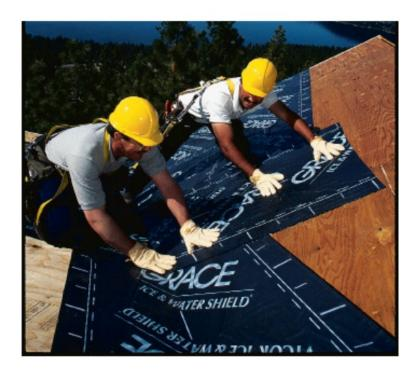
**Dual barrier protection** – Rubberised asphalt and polyethylene are combined to form two waterproofing barriers providing maximum protection.
